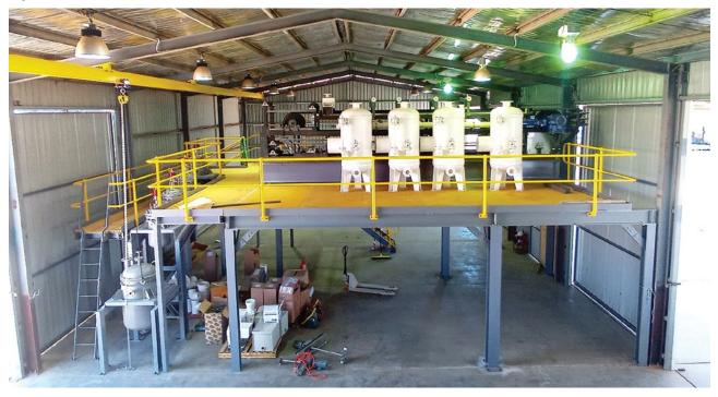
Figure 2 - Pilot Plant Progress - installed autoclave reactors in foreground
