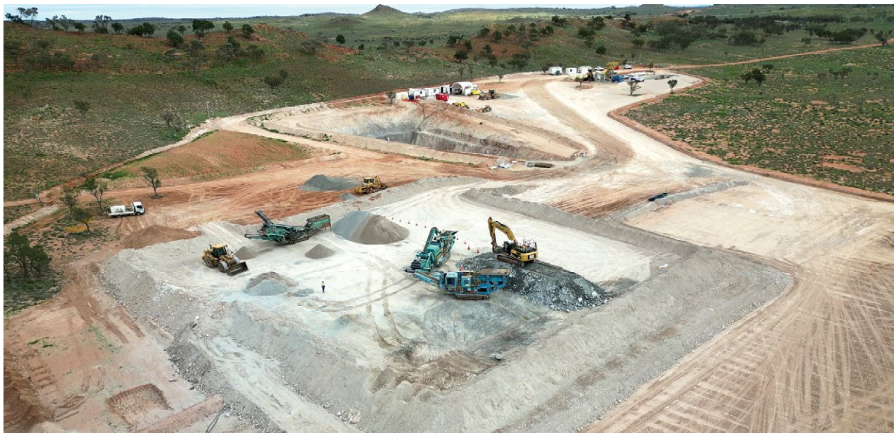
Figure 6 – Multi-stage crushing plant processing ore stockpile in preparation for milling.
