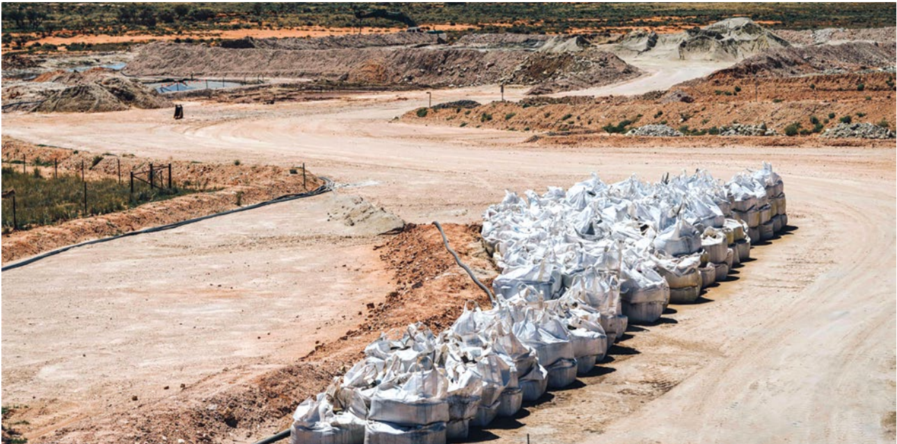
Figure 1 – Bags of concentrate at the Broken Hill Cobalt Project awaiting transport to the Demonstration Plant in Broken Hill township.
