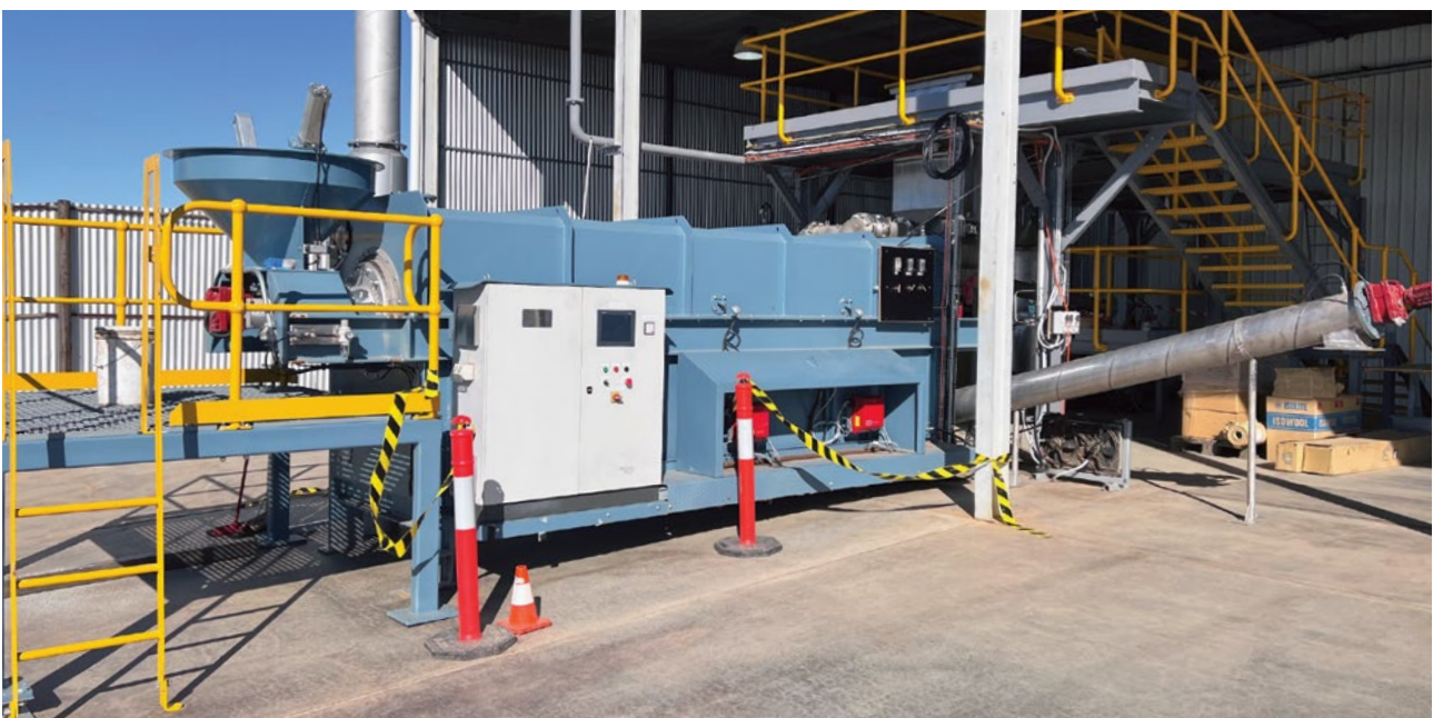
Figure 2 – Demonstration Plant Kiln to convert pyrite into pyrrhotite and elemental sulphur.
