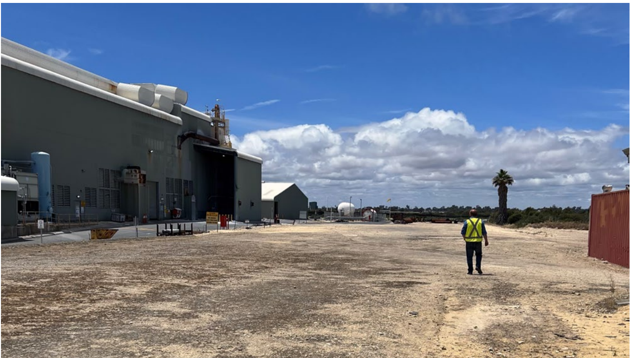
Figure 3 – Proposed refinery site adjacent to Doral Fused Materials operation
