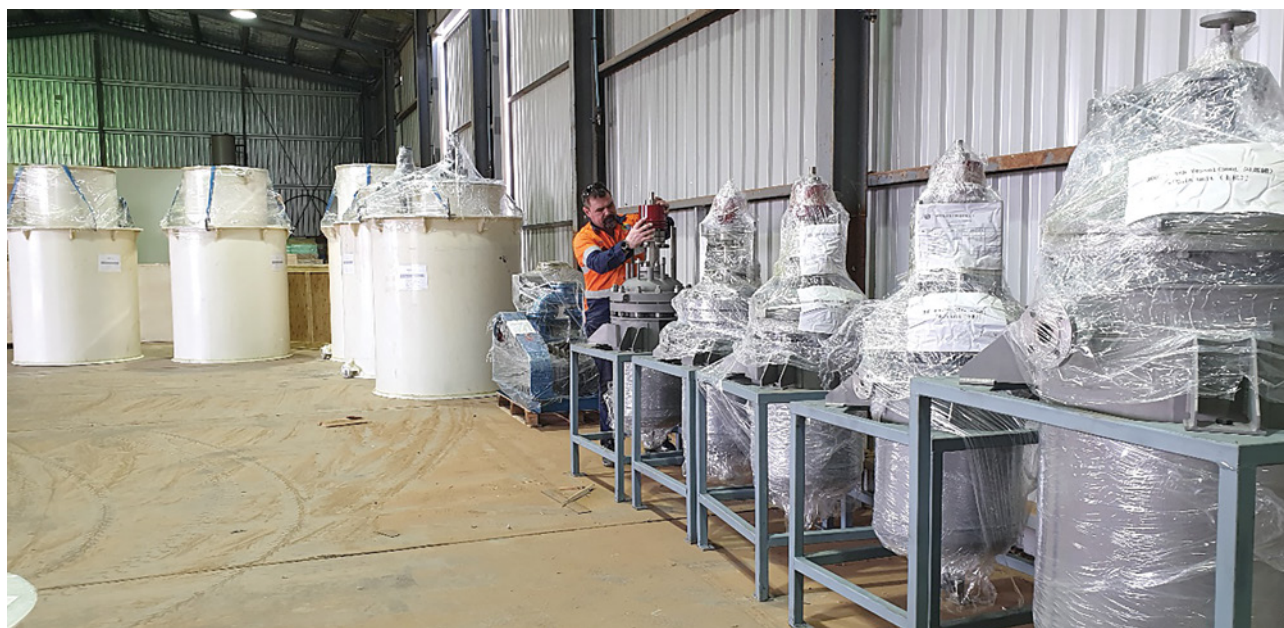
Figure 3 – COB Pilot Plant – Leaching Circuit Equipment received by Adam Randall (Plant Manager)
