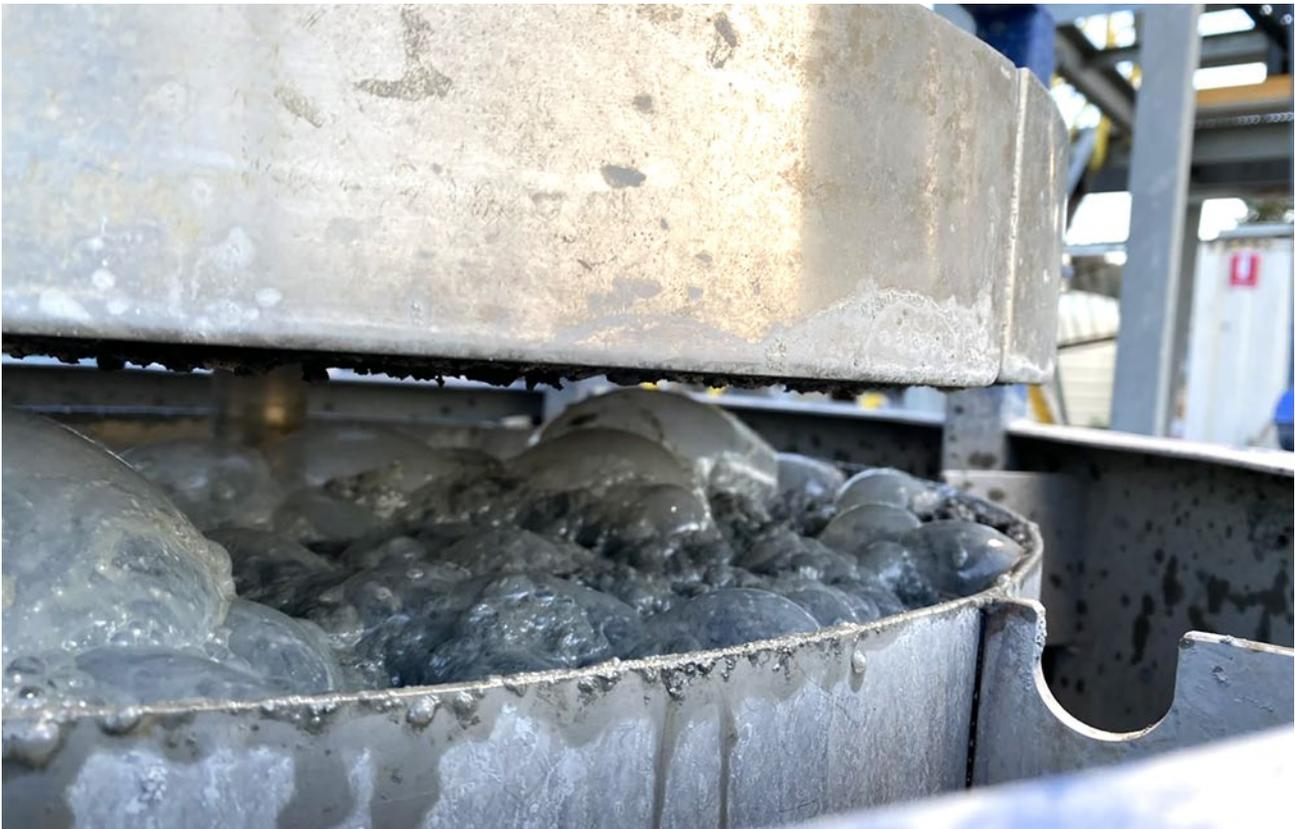
Figure 5 – Dewatering cyclone for final tailings
