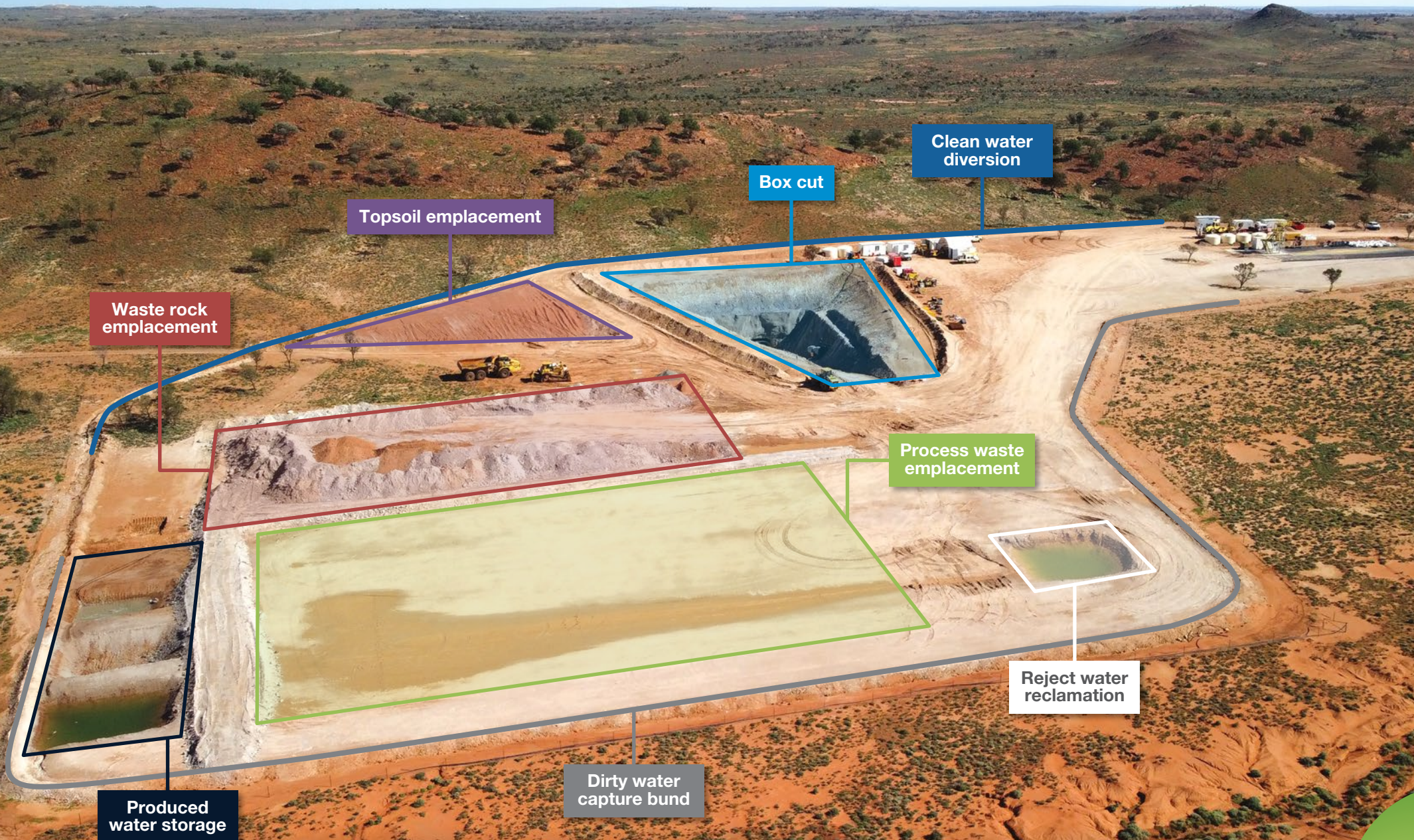
Figure 1: Bulk sample showing environmental controls – the underground box cut, waste and ore storage pads
